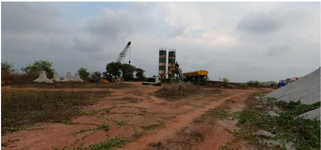
Figure 3: Halted Port Construction
