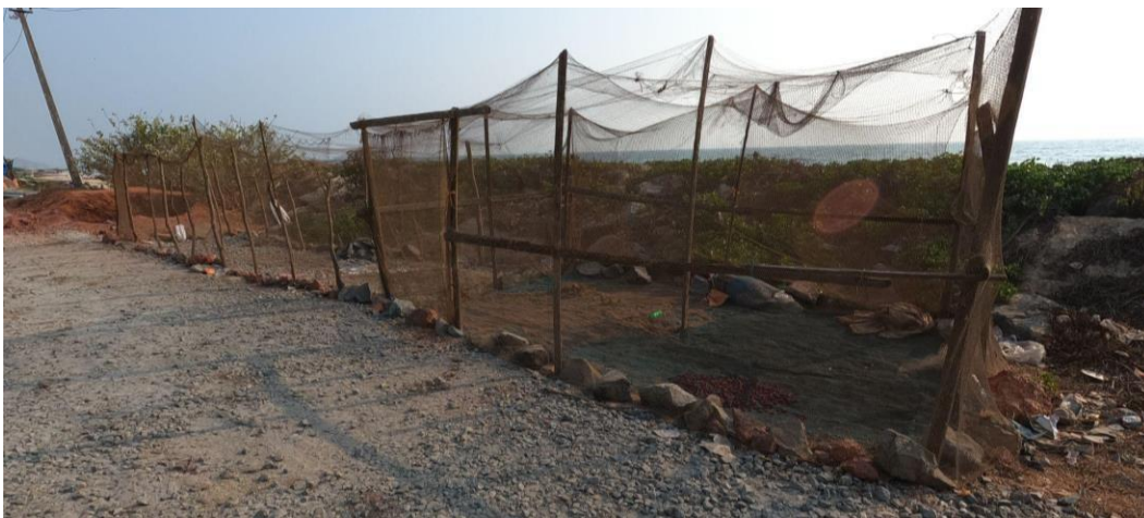
Figure 12: Fish drying on under construction road
