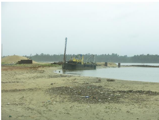
c. Construction activity along the eastern boundary of the port
